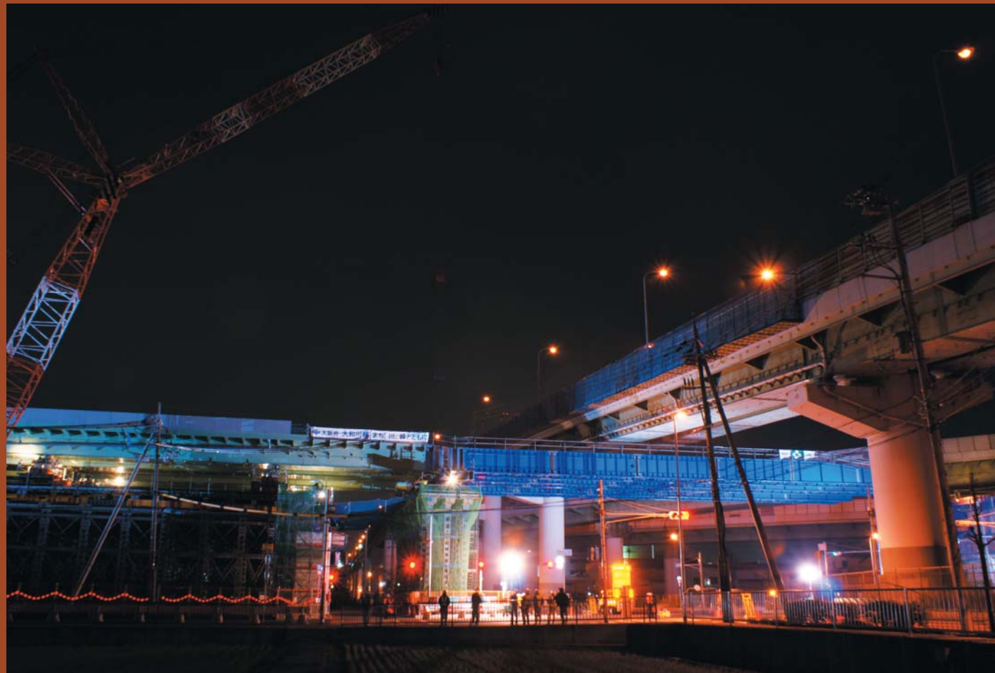
国道309号の送り出し架設施工状況 Bridge-erection-by-launchine on Route 309
