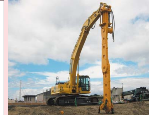
WILL工法施工機械 Construction machinery equipped for the WILL method
