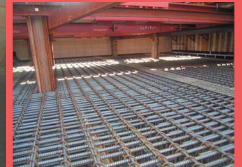
配筋状況 Arrangement of reinforcing bar
