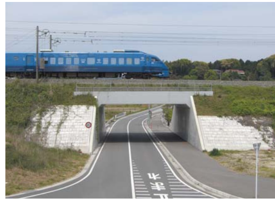
完成事例 (JR鹿児島本線・海老津) View of completed construction (Ebitsu, JR Kagoshima Main Line)
