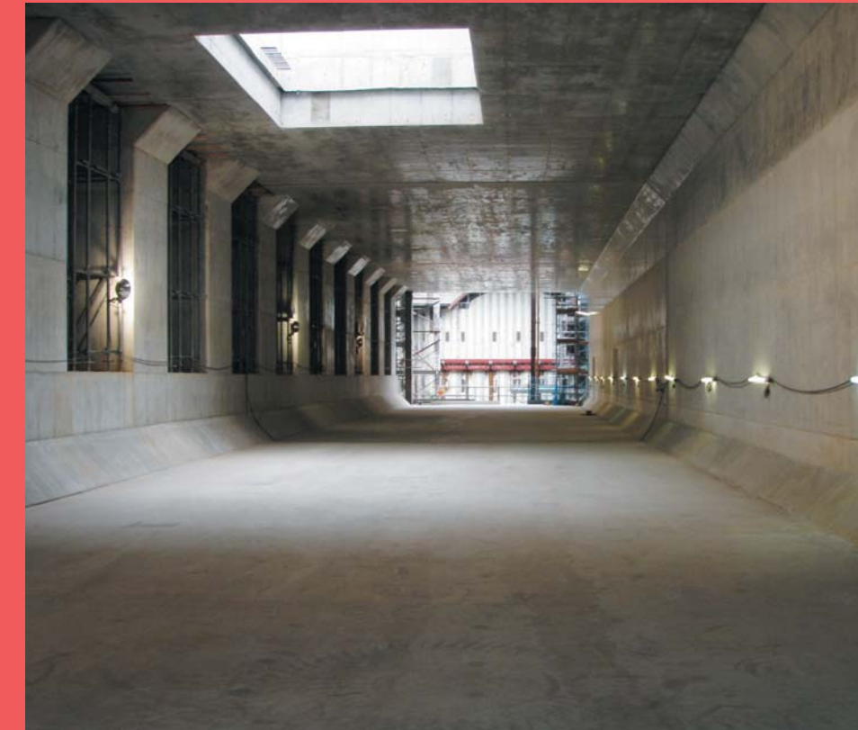
函体の完成状況例 Completion of cut-and-cover tunnel structure
