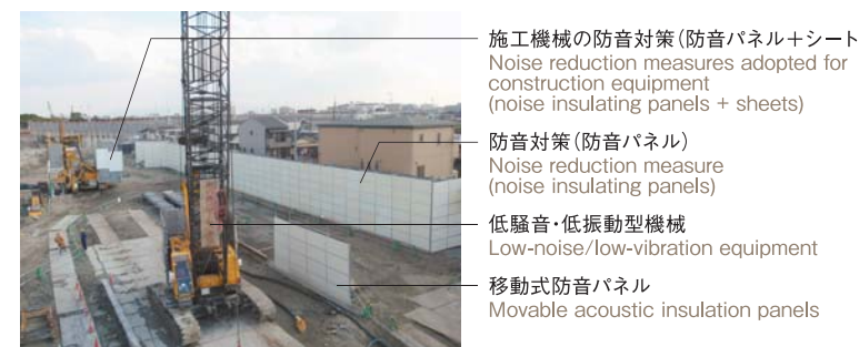
住居近接地区における騒音・振動対策 Noise/vibration reduction measures adopted for the benefit of residents of the adjacent community
