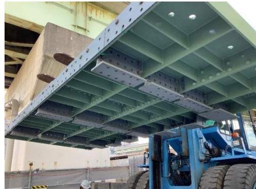
(c) 鋳鉄床版の架設
